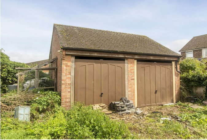
Brick constructed double garage with two up and over doors.
