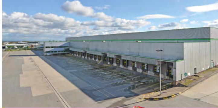
28 DOCK LEVEL LOADING DOORS
