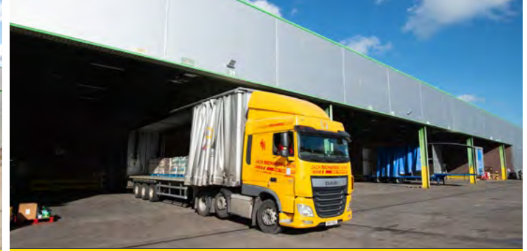
6 DRIVE IN LOADING DOORS
