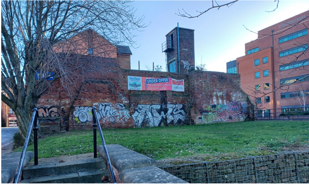
5 // Locally Listed Cocker Brother Cementation Furnace
