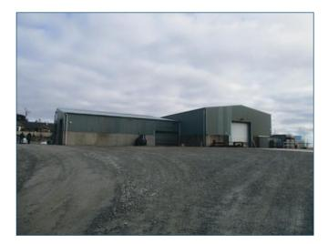
Office and staff accommodation is contained within a single storey rendered blockwork extension with profile clad roof.
