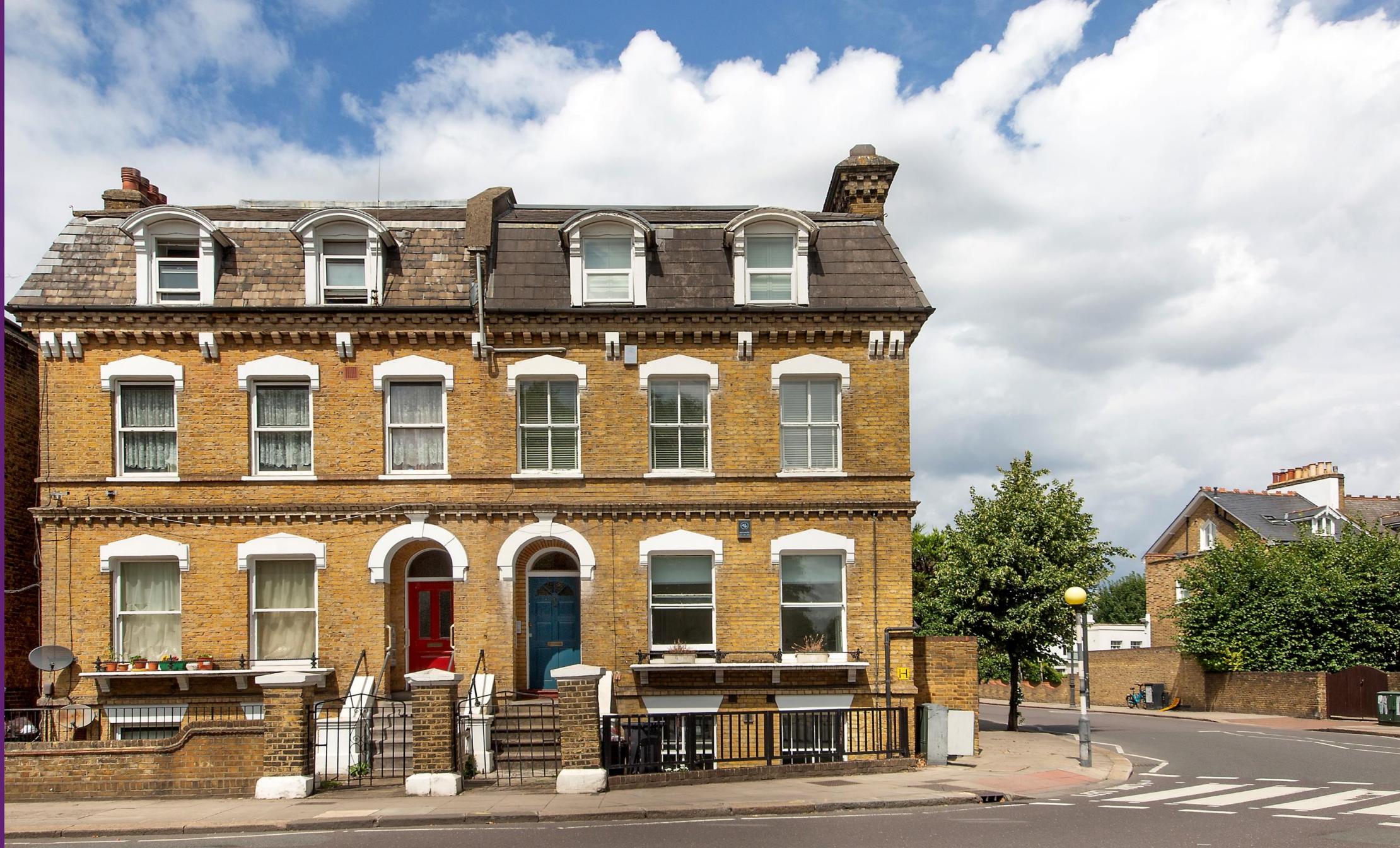
North Side Wandsworth Common London, SW18
