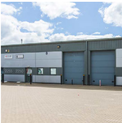
2200 1,100 sq ft to 6,500 sq ft 16 modern steel portal frame industrial units arranged in three terraces, facing a shared yard. The units include standard glass fronted door, 4m high roller shutter door leading to ground floor workshop and WC and first floor mezzanine. Minimum height to underside of eaves 4m, yard depth 20m.
