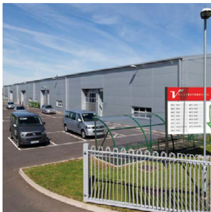
BUCKINGHAM ROAD 5,000 sq ft to 13,000 sq ft Located within the Enterprise Zone. 15 light industrial units arranged in three terraces, constructed of steel portal frame with profile metal clad walls. At ground floor level units include warehouse area with 6m to underside of eaves, fitted reception, office, toilet and stairs to first floor mezzanine. All units benefit from an electrically operated surface level loading door, leading to a yard area and parking.
