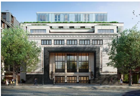
Holland Park Gate, W8
