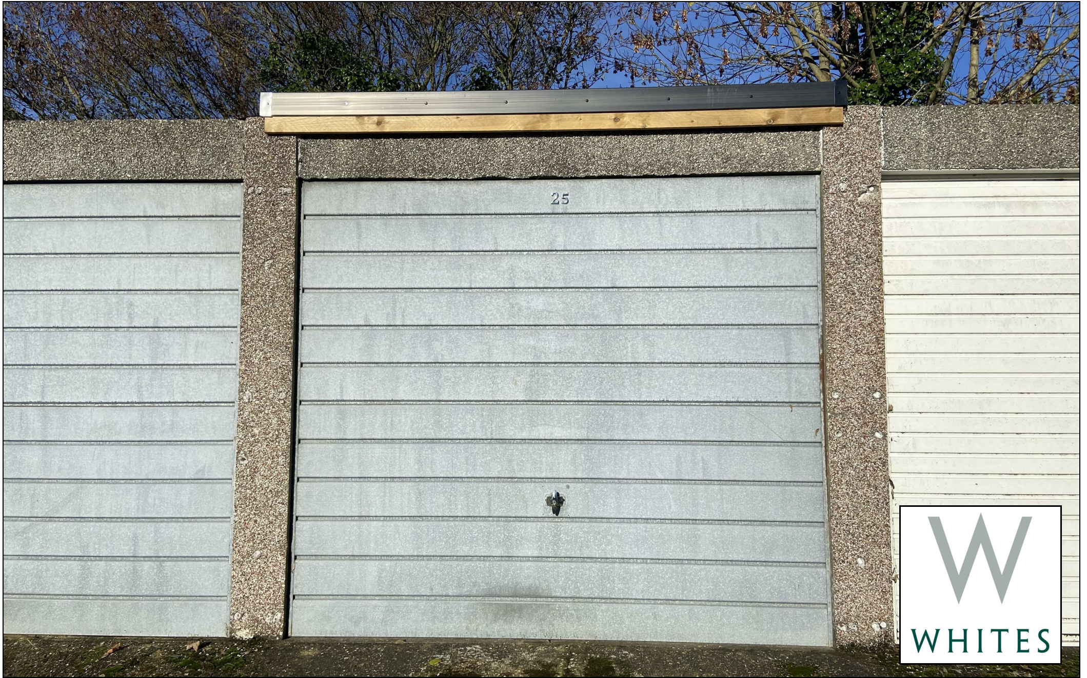
Garage 25 St Francis Road, Salisbury, SP1 3QP
