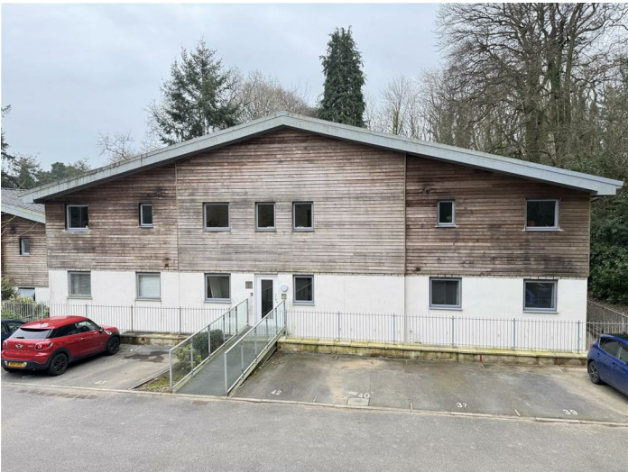
The property benefits from use of the communal gardens within the complex, as well as allocated parking space and communal bin/recycling store. The property also benefits from having private access to Duporth Beach.
