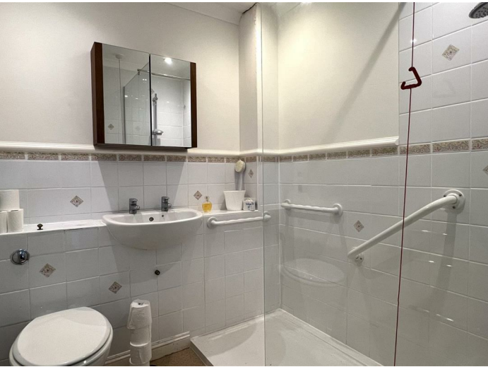
A re-fitted suite comprising of low level WC, hand basin and shower. Part tiled wall surround recessed spotlighting and ceiling extractor.
