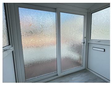
UPVC double glazed sliding patio door with obscure glazing allows external access into front porch. With matching sealed glazed units to right hand side of the front door and matching window to the right and left elevations. Wood effect laminate flooring. UPVC clad ceiling. UPVC double glazed door with matching obscured glazing allows further access into kitchen.
