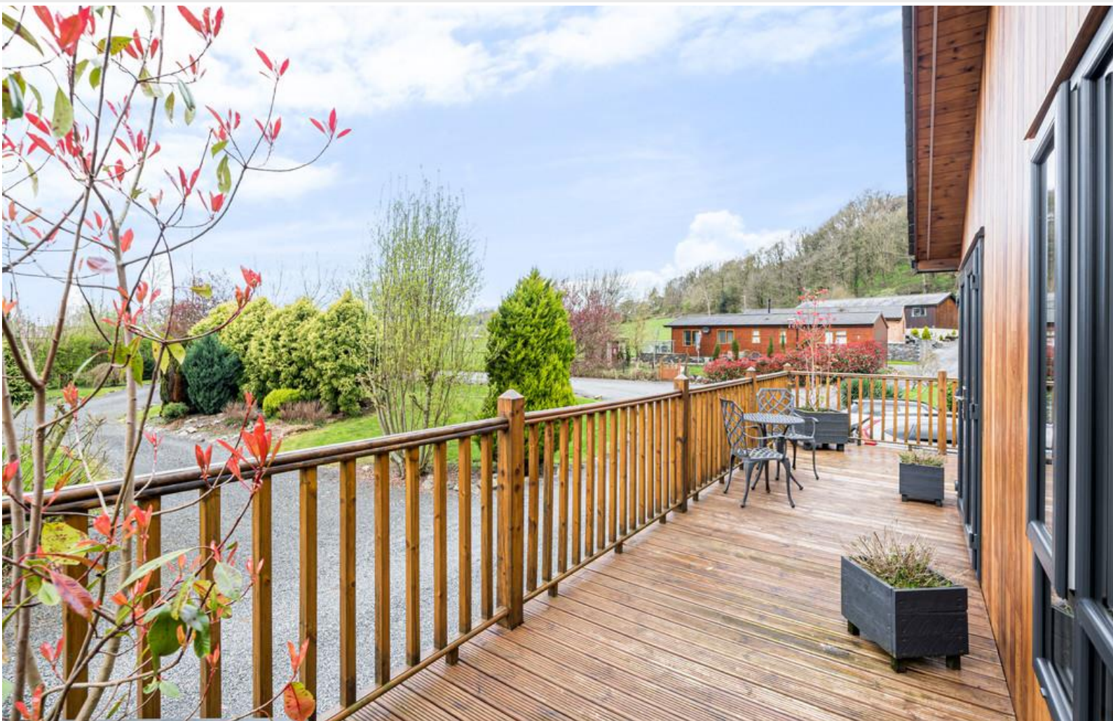
Front Balcony Decking
