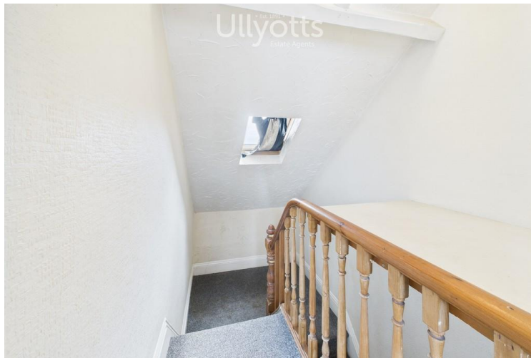
Second Floor Landing
