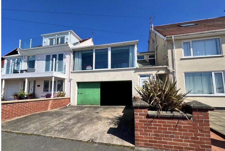
Front Elevation - Right Hand Side Garage Does Not belong to this property
