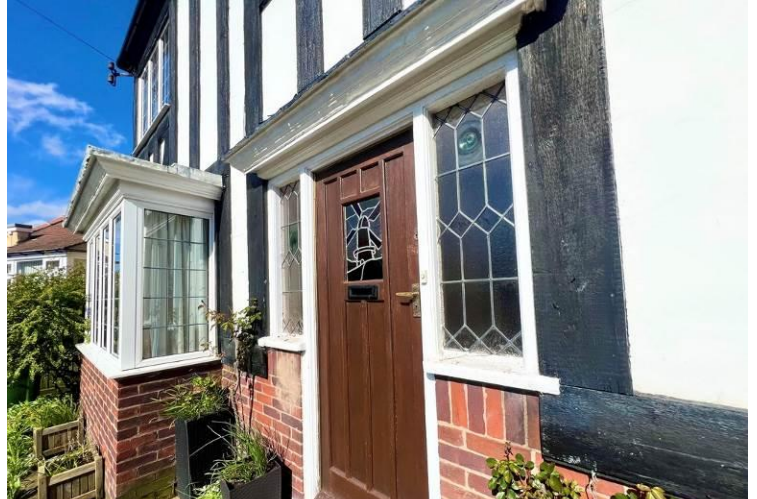
Front Elevation Close Up
