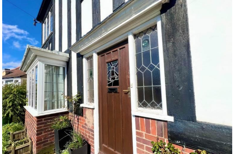
Front Elevation Close Up
