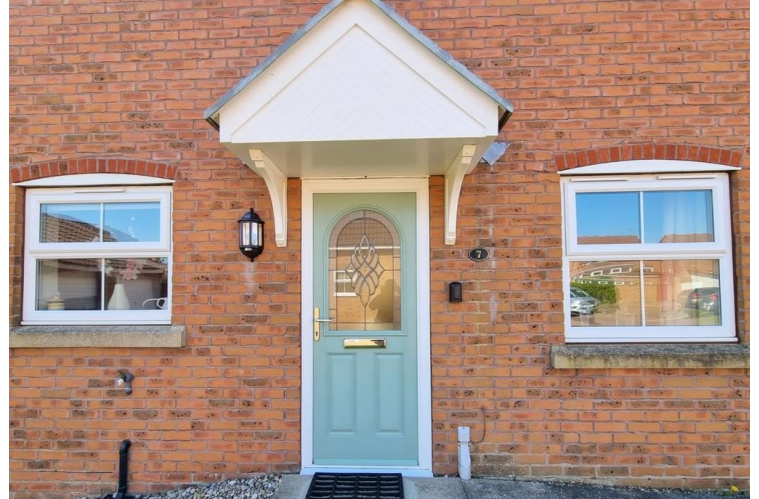
Front Elevation Close Up
