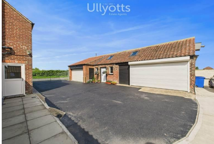
Garages and workshop
