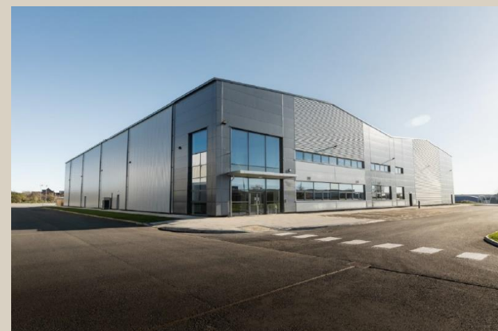
Intersect 19 recently completed in North Tyneside by UK Land
