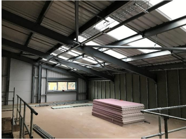
First floor of Unit 5 under construction
