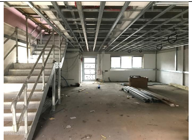
Internal ground floor of Unit 4
