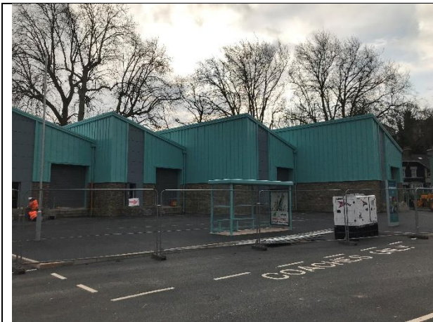
Units 2, 3, 4 & 5 from the front
