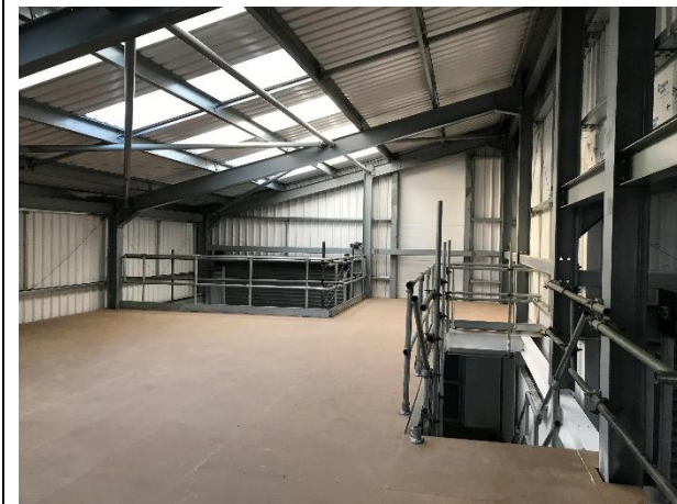
First floor of Unit 5 under construction
