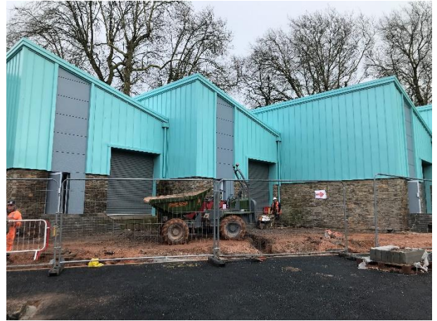
Front of units 2, 3 and 4 under construction
