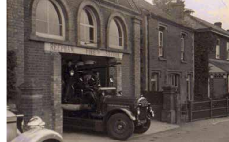
Reepham Fire Station, 1936.
