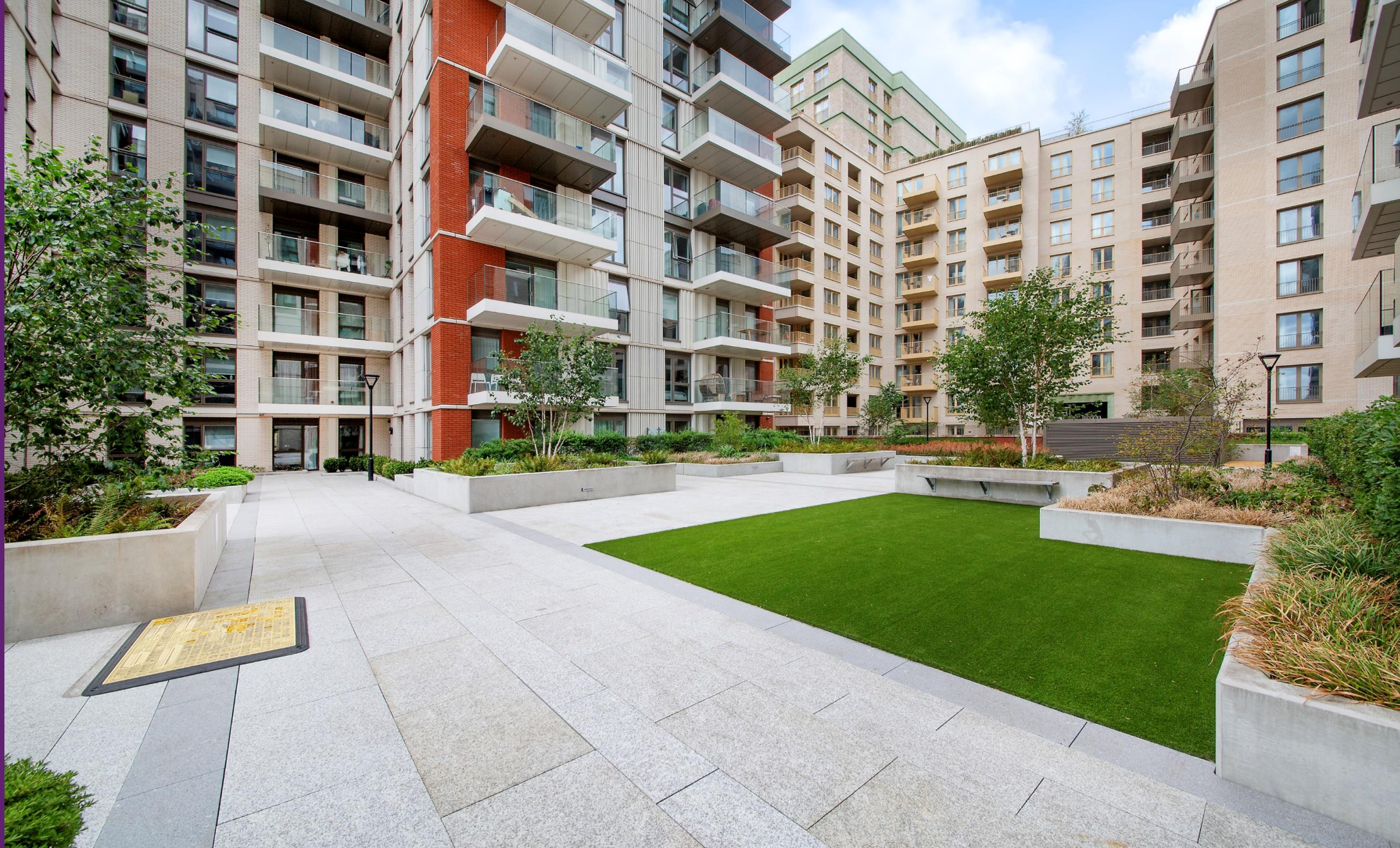
Montrose Building Lexington Building, SW11
