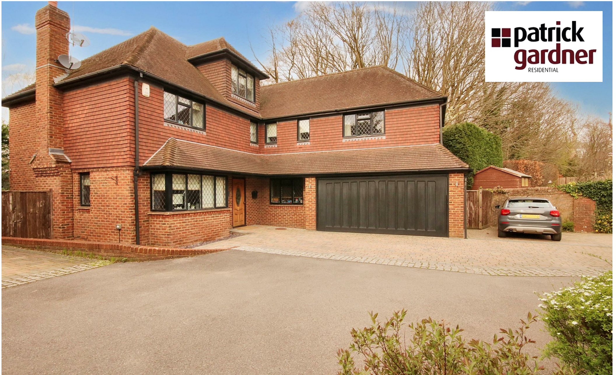
Mill Bank Cottage, 7 Park Lane, Ashted, Surrey, KT21 1DW
