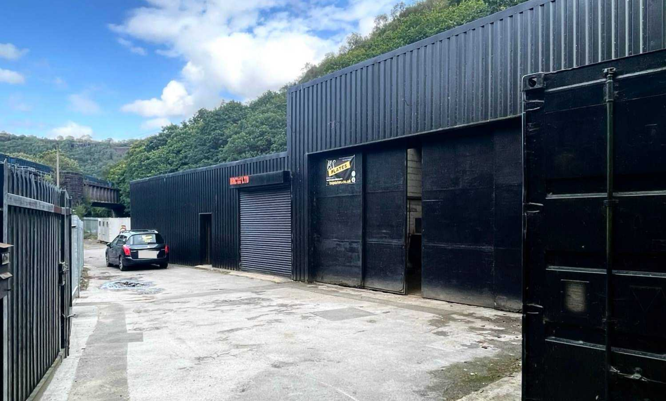
Whiteley Arches Garage, Calderside Hebden Bridge
