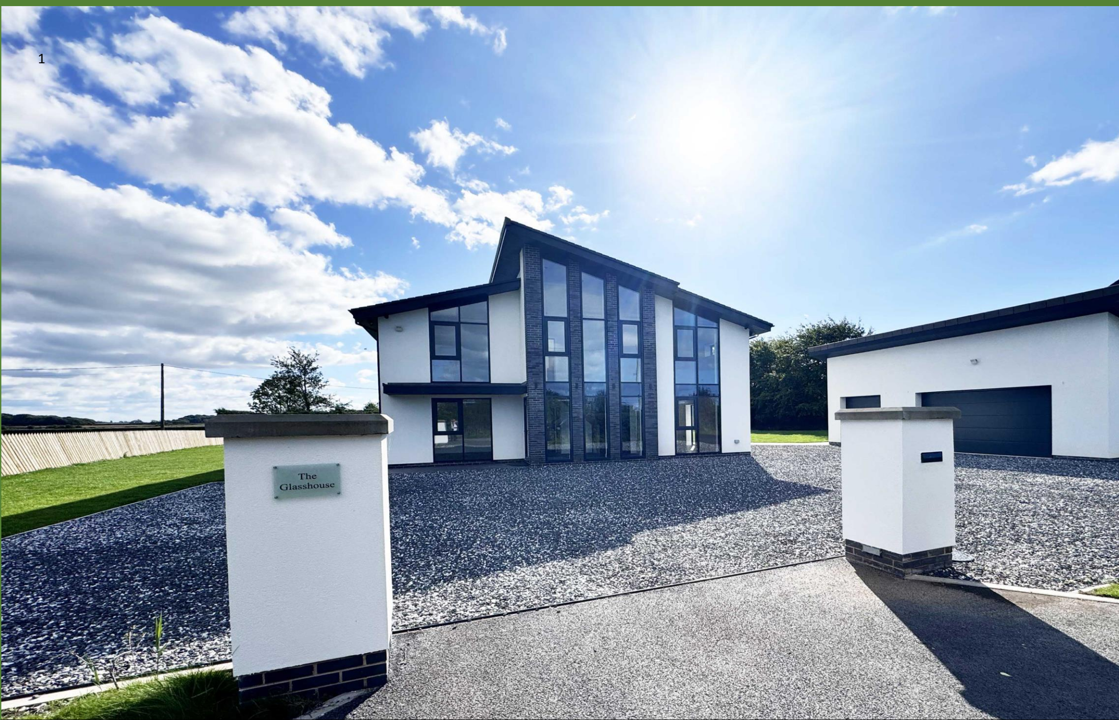
THE GLASSHOUSE, PUDDLE HOUSE LANE, FY6 8LB
