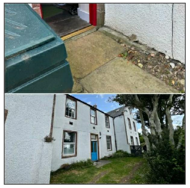
External ground level was high in areas in relation to internal floor level which may lead to water penetration.
