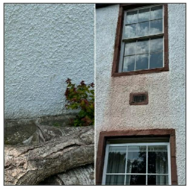
Staining indicative of exessive water running down the render was noted which may lead to water penetration through the walls, failure to repair this could result in spoiling of internal wall fabrics and fungal decay to concealed timbers.
