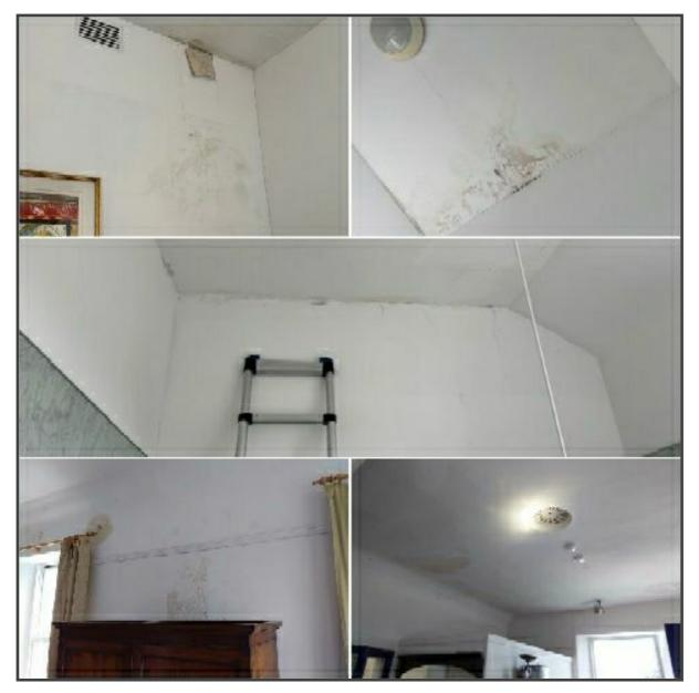
Our inspection of the internal ceiling & wall surfaces of the property was carried out by a visual inspection and by the use of an electrical conductivity meter; As highlighted in the first three sets of collage photos above, this indicated penetrating damp to be present in the ceiling of the Hallway & the walls of the Lounge, Kitchen and rear left Bedroom designated for treatment on our enclosed sketch plan.
