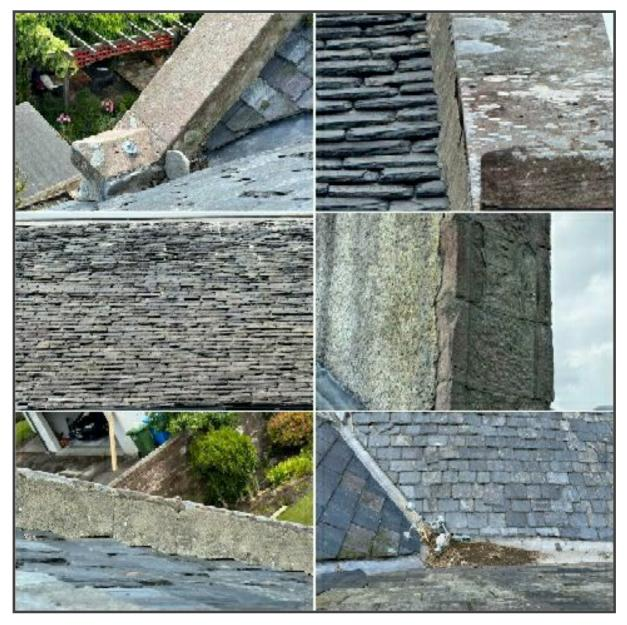
Defective cement work noted to the roof coverings which can lead to water penetration, failure to repair these could result in spoiling of internal wall fabrics and fungal decay to concealed timbers.
