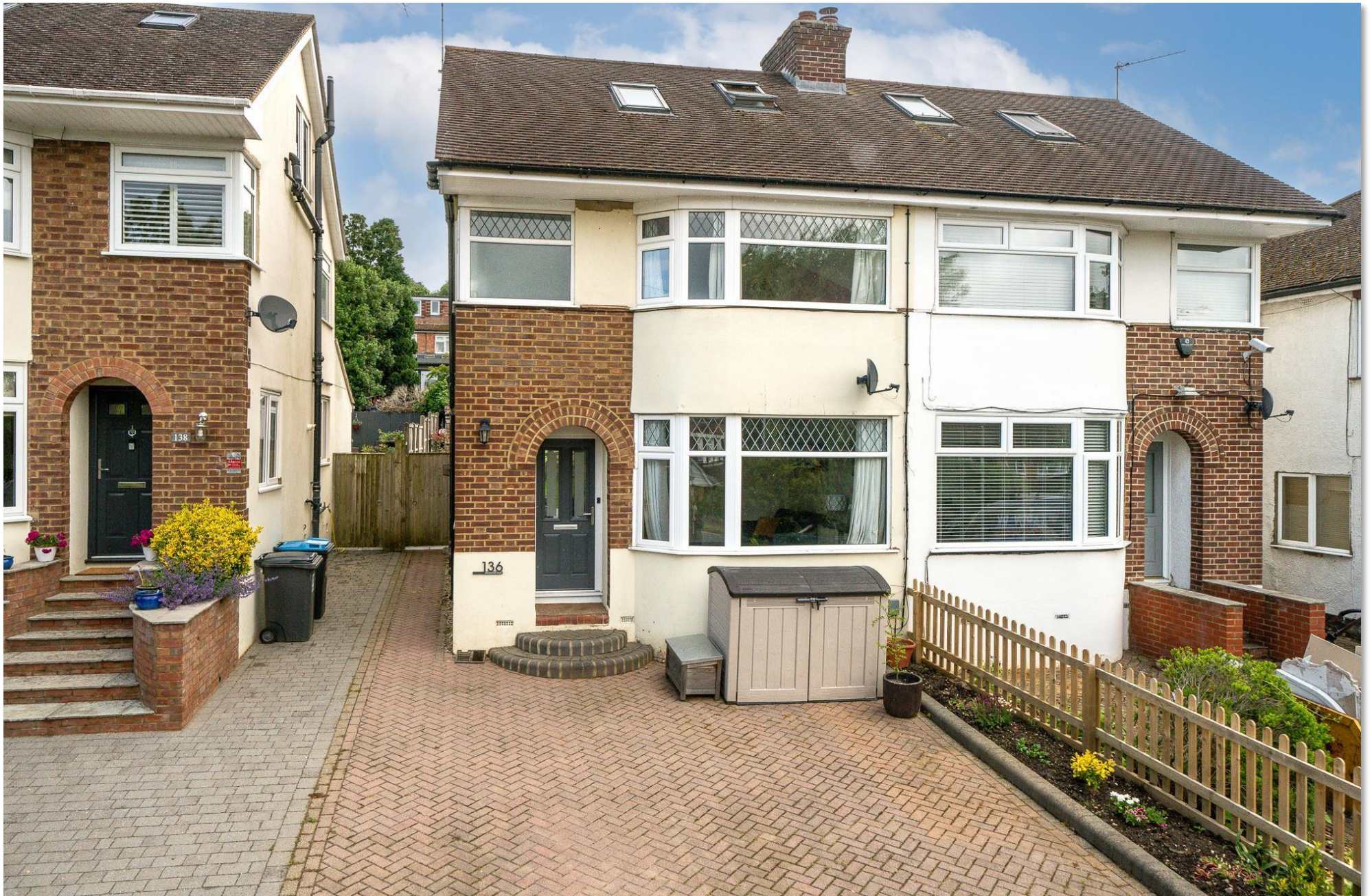
Bridgewater Road, BERKHAMSTED HP4 1EE
