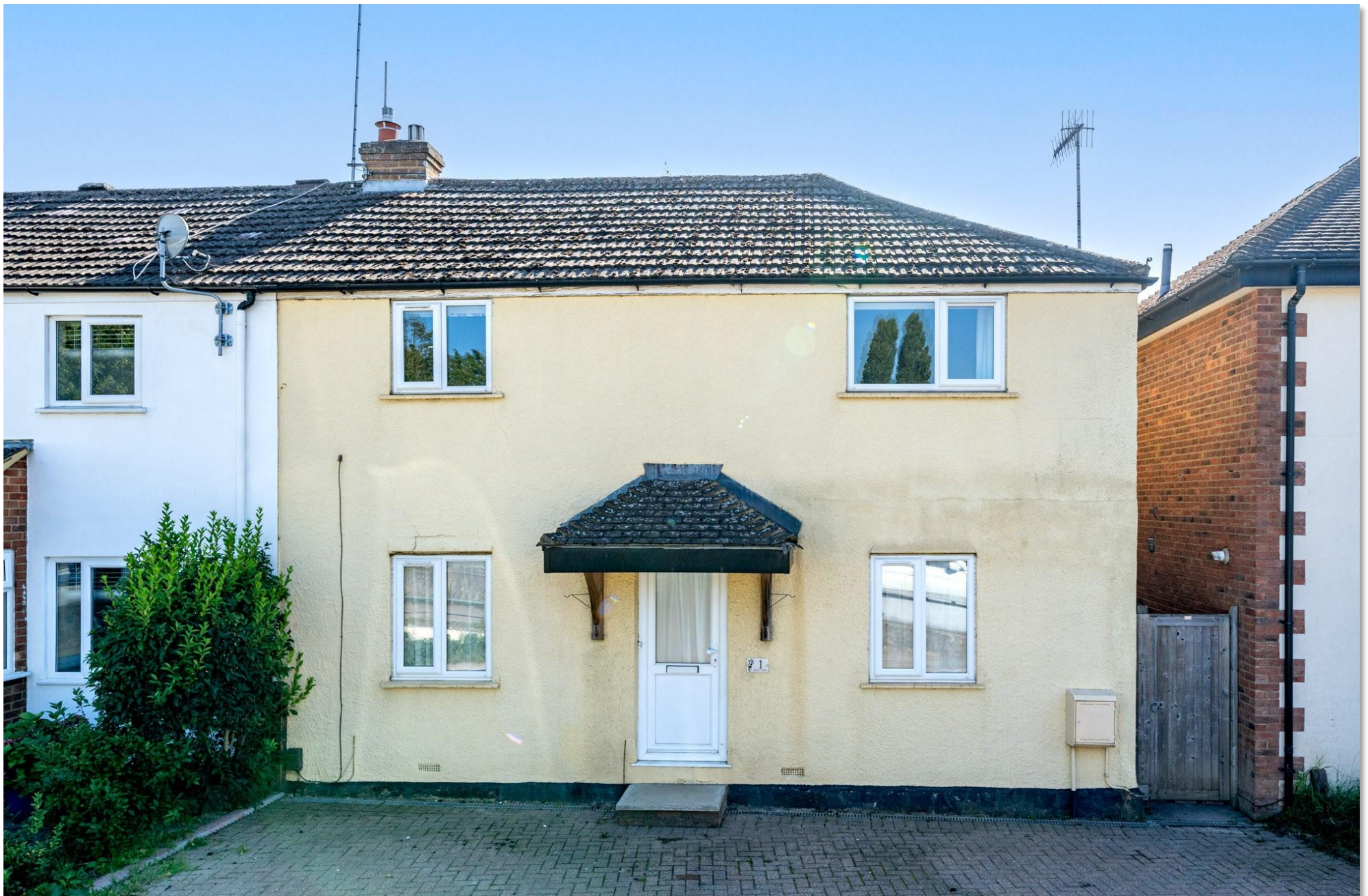
Billet Lane, Berkhamsted HP4 1DP
