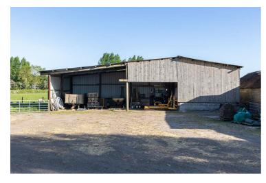
Timber pole with part concrete block walls, steel box profile and timber cladding, steel box profile and corrugated steel roof, earth floor and floodlight.
