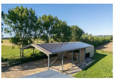
Modern 6 bay steel portal frame Straw Barn with fibre cement roof incorporating solar panels, 6.70m to eaves, concrete/hardcore floor, concrete panel walls and Yorkshire Board cladding and access gates to the two east bays and adjoining solar panel inverters with power supply.
