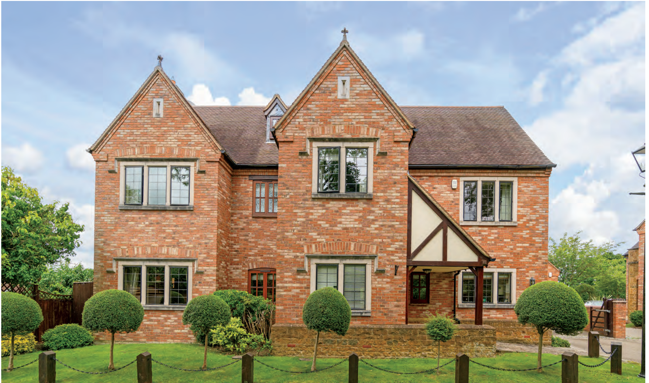
The Old Pavilion Main Street | Flecknoe | Warwickshire | CV23 8AT
