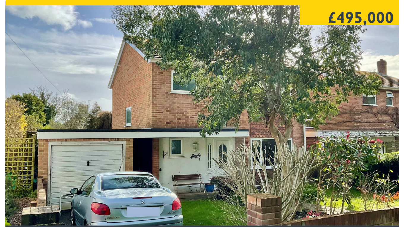
Shingles | Jarvist Place, Kingsdown, Deal CT14 8AL
