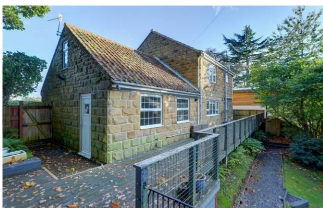
Rear Elevation and Walkway
