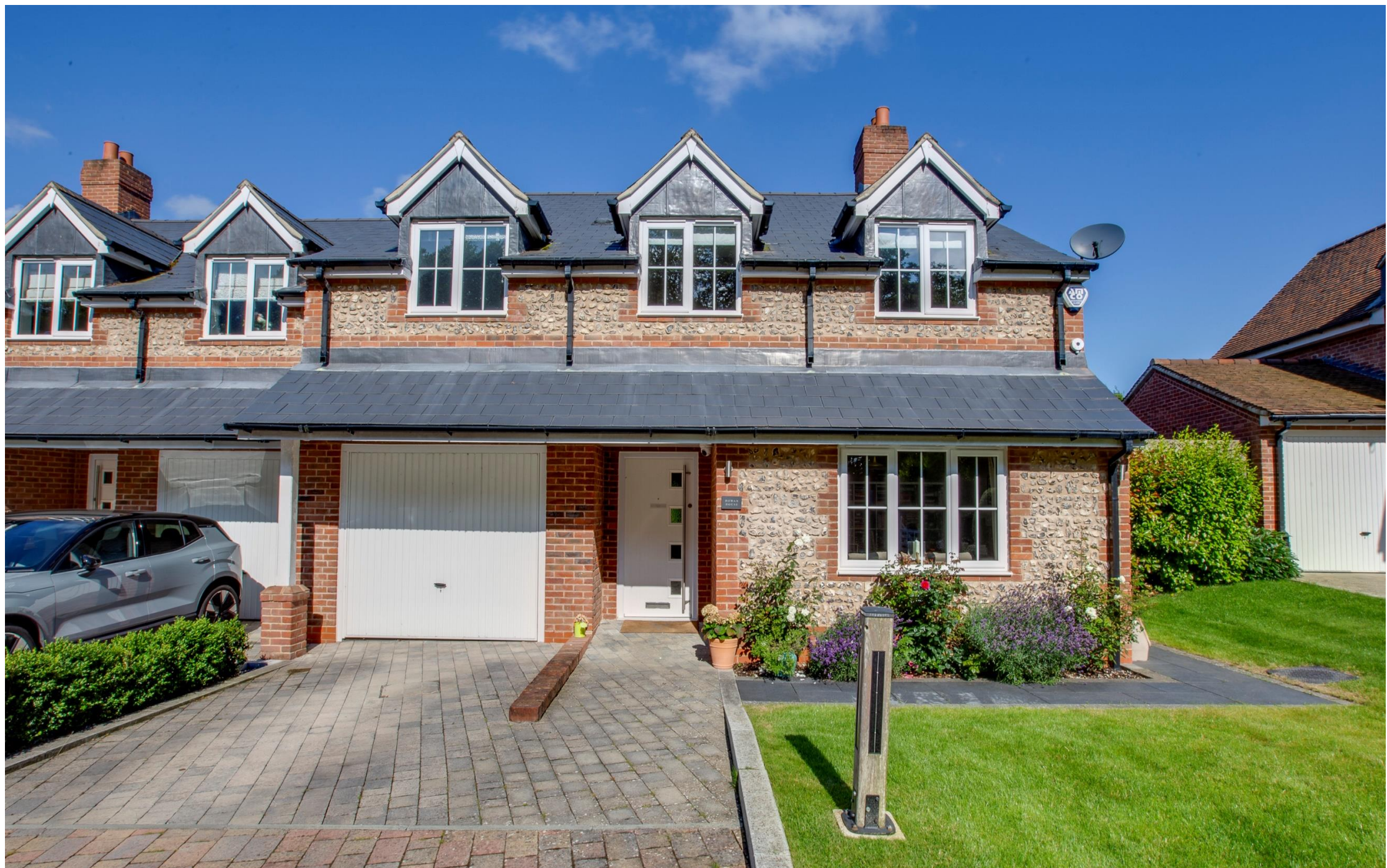
Rowan House Hammersley Lane
