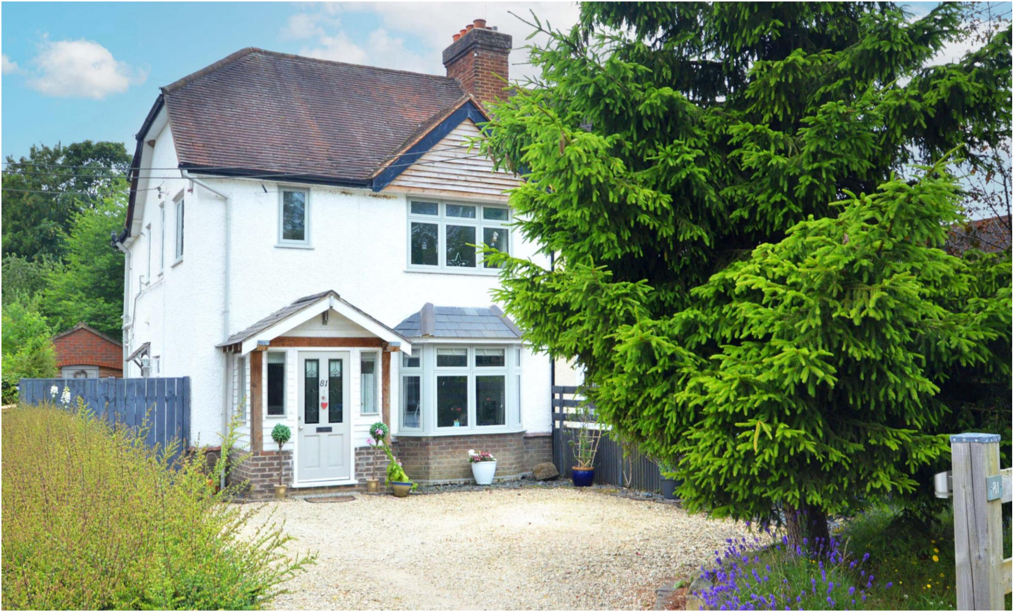
Summerleys Road Princes Risborough
