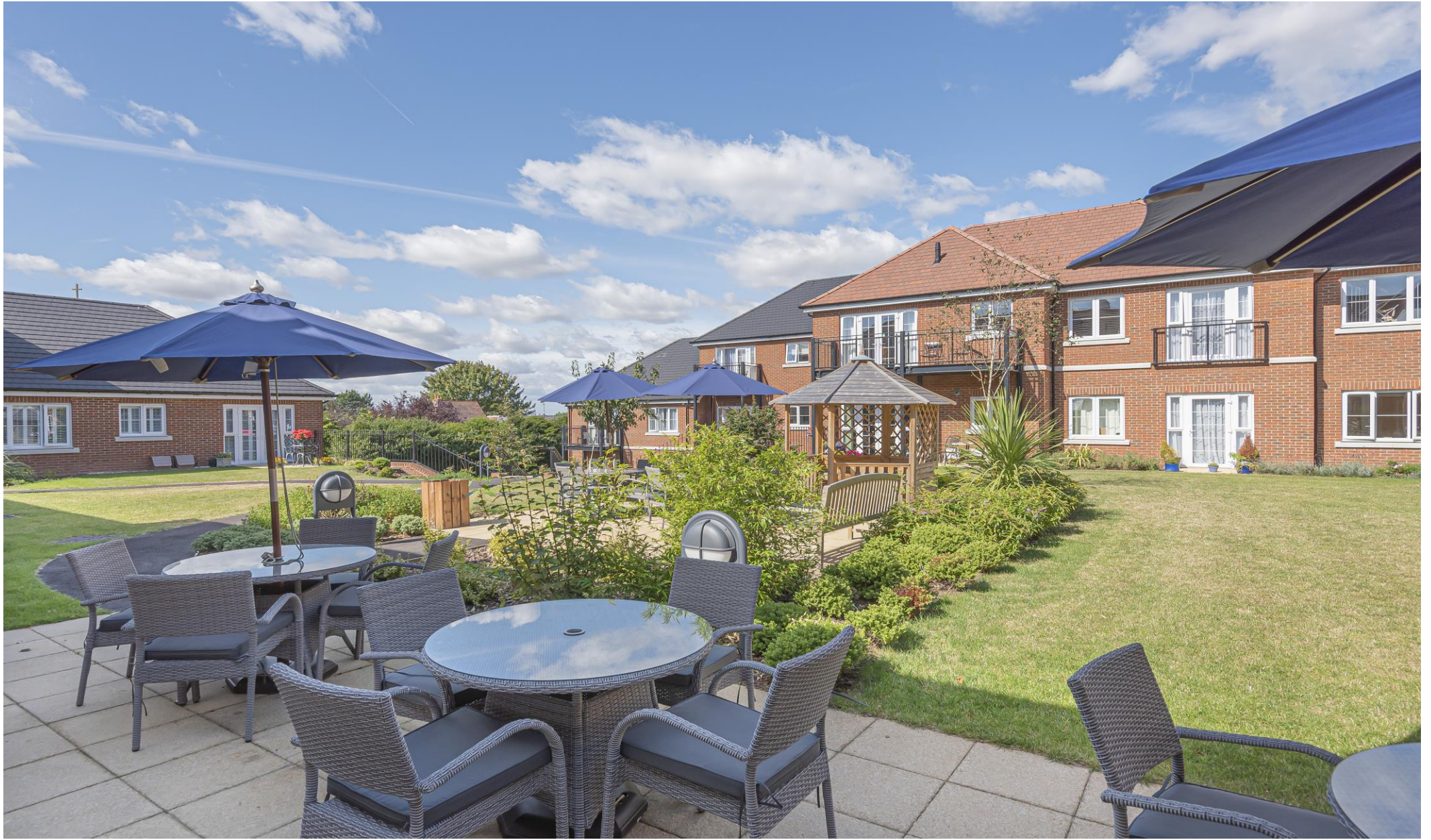
42 Eaves Court Princes Risborough
