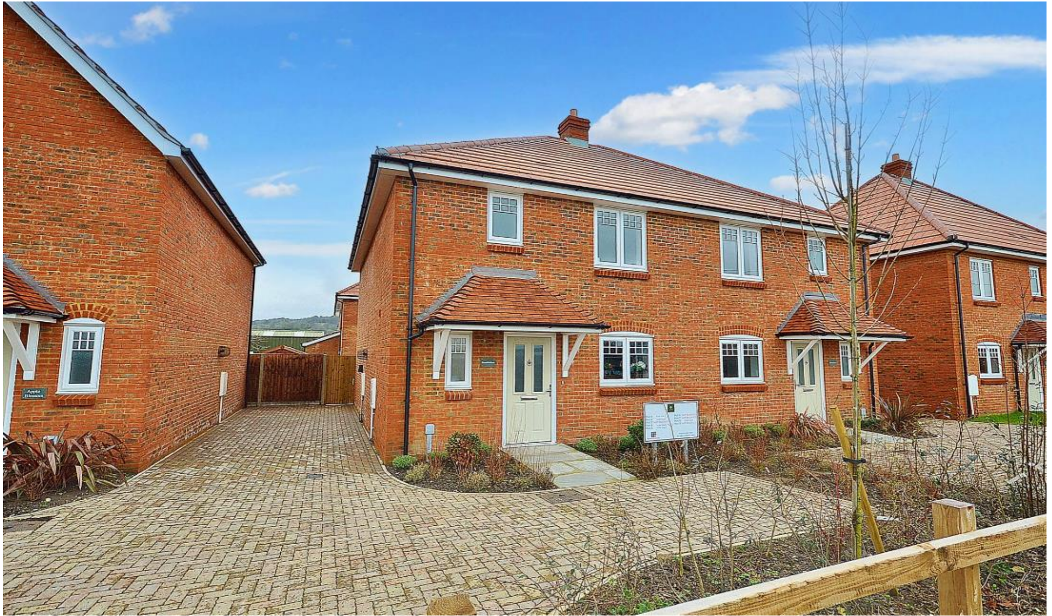
Plot 2, Pippin Place Grove Lane, Great Kimble
