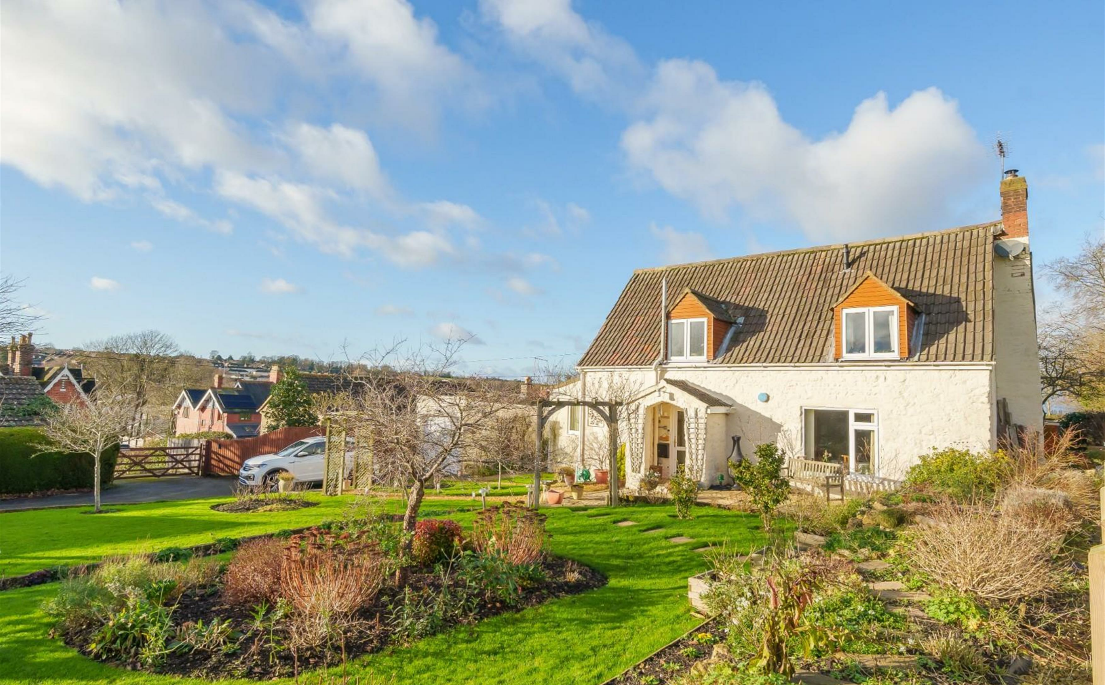
Mill Cottage, 3 Hopton Road, Dursley GL11 5NZ
