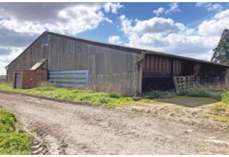
To the west of the site is a single storey open-fronted cart shed  $10.76 \,\mathrm{m} \times 7.41 \,\mathrm{m}$  of timber framed construction partially enclosed with timber feather edged boards under a box profile steel sheet roof.
