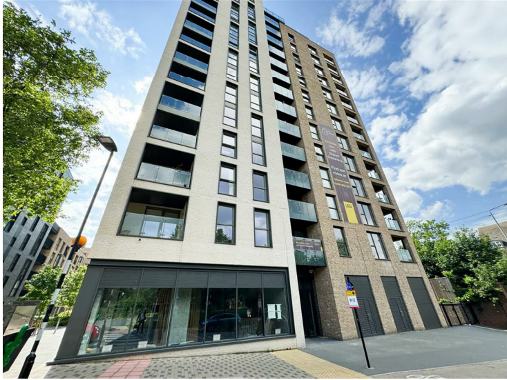
Front Of Building
