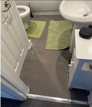
22-11-2024 10:58 / Bathroom Flooring / 6t9fjszck
