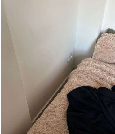
22-11-2024 10:59 / Bedroom Walls Ceilings / Tv1b88i4q
