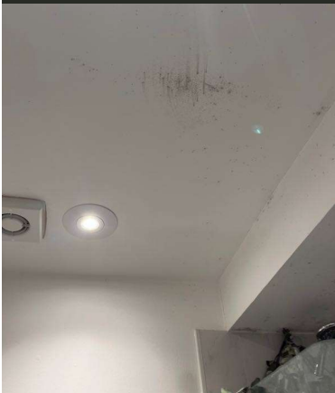
22-11-2024 10:58 / Bathroom Walls Ceilings / 69omdtpgn
