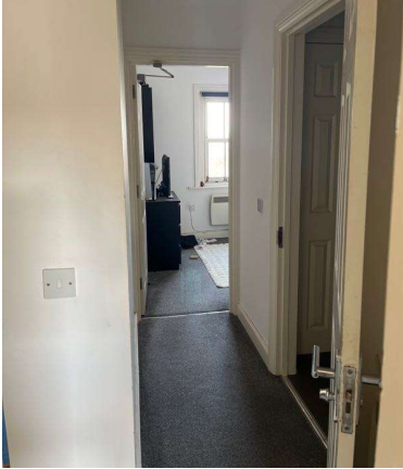
22-11-2024 10:57 / Walls Ceilings / Hw3z2qofb
