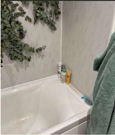
22-11-2024 10:58 / Tiles Grout / Cdmpam4z7
