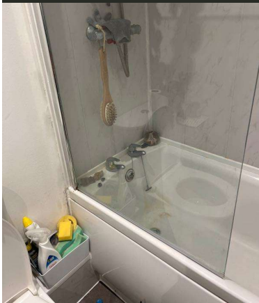
22-11-2024 10:58 / Tiles Grout / 11ly1e4f6
