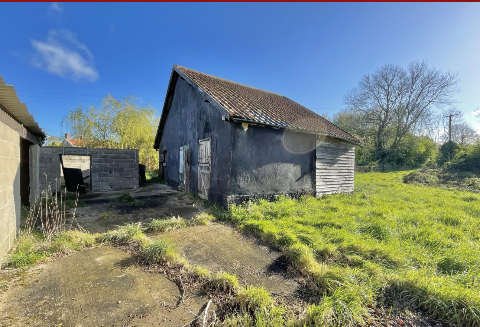
Town Farm Barn The Street, Ovington, IP25 6RT
