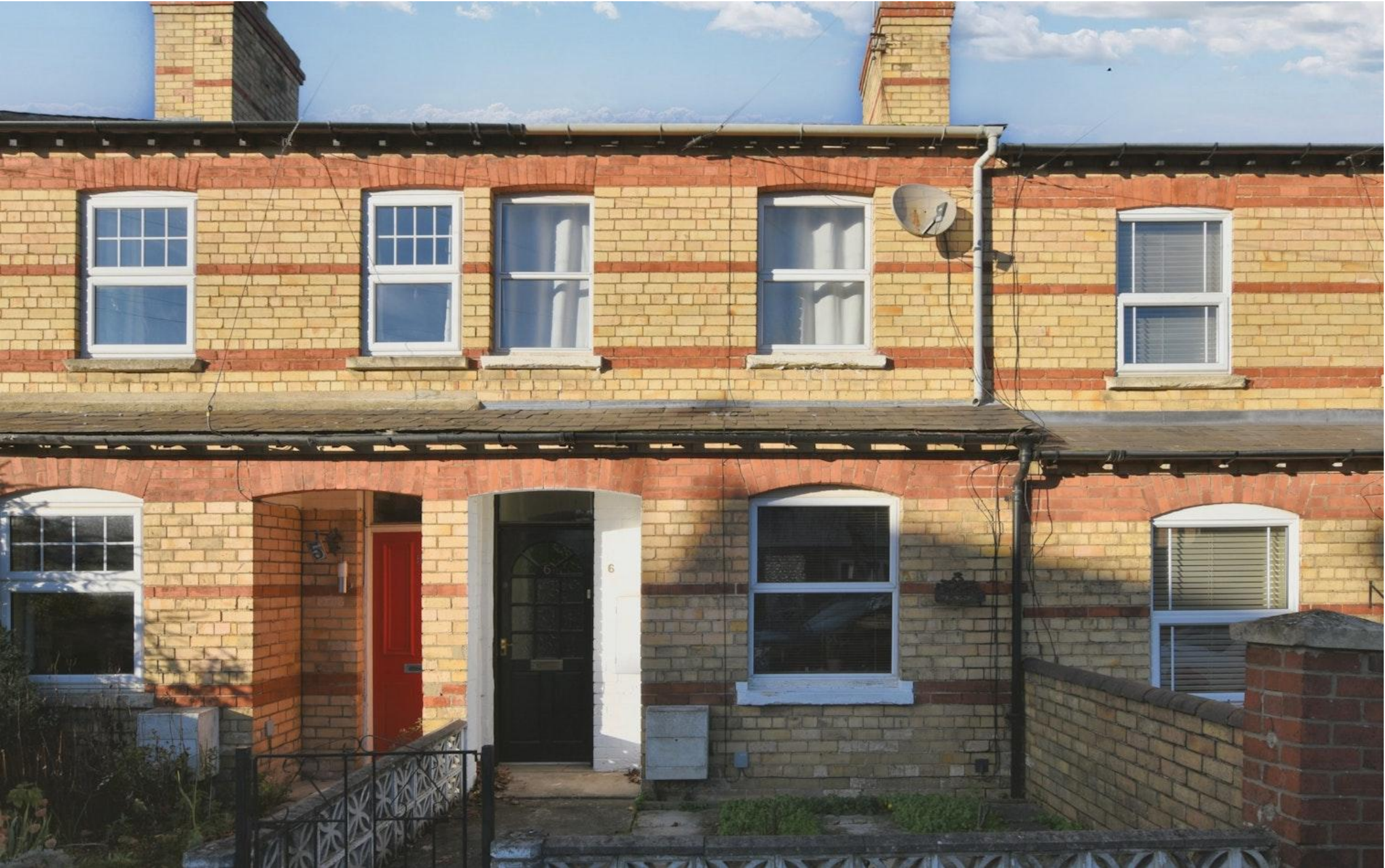
South View Terrace, Stamford
