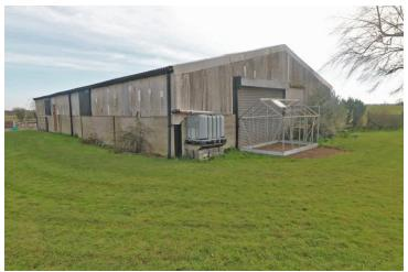
PORTAL FRAME CONSTRUCTION:45' 2"  $\times$  25' 11" (13.771m  $\times$  7.900m) Doors to both ends of the building with stalls. Hard standing floor. Power and water.
