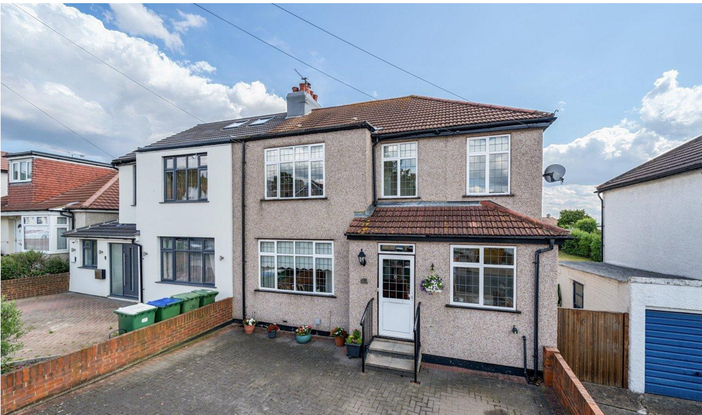
Boundary Road, Sidcup, DA15 Approximate Area = 1351 sq ft / 125.5 sq m For identification only - Not to scale
