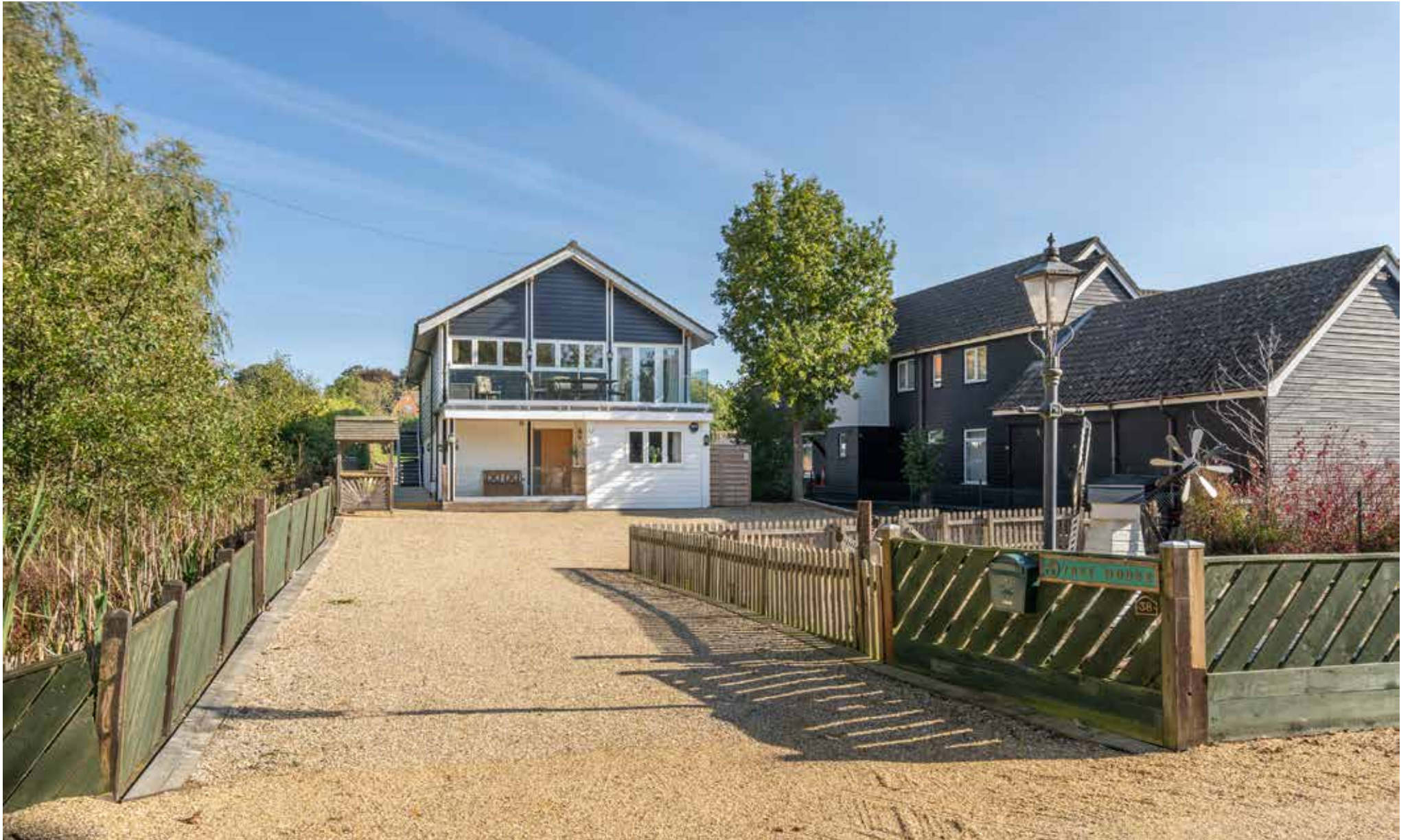
Tree House 38 Ropes Hill Dyke | Horning | Norfolk | NR12 8JS
