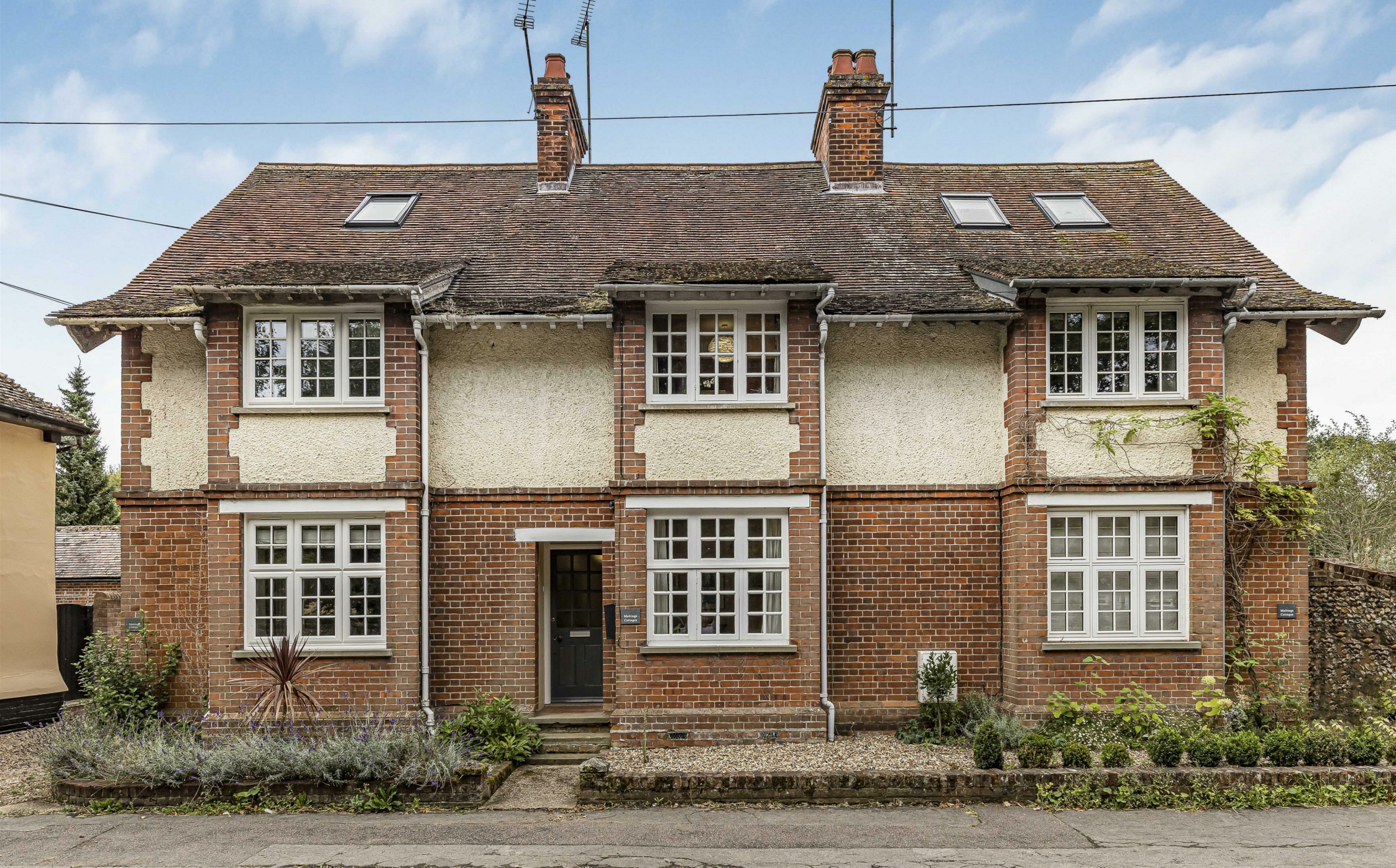
Maltings Cottage, Bartlow, CB21 4PW
