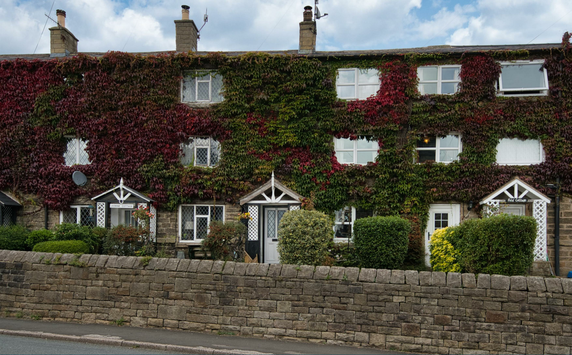
Victoria Cottage, Ashopton Road, Bamford, Derbyshire, S33 0DB
