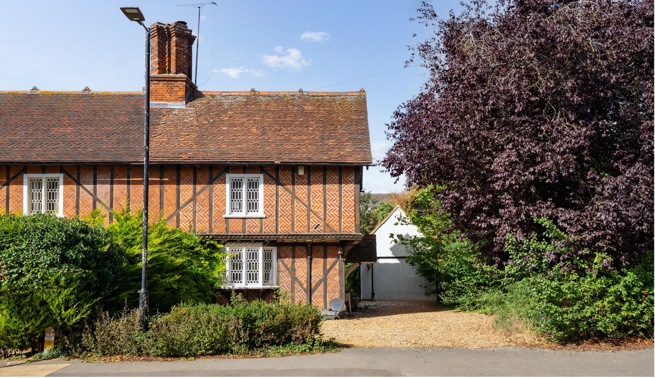
Pond Cross Cottage, High Street CB11 3PQ
