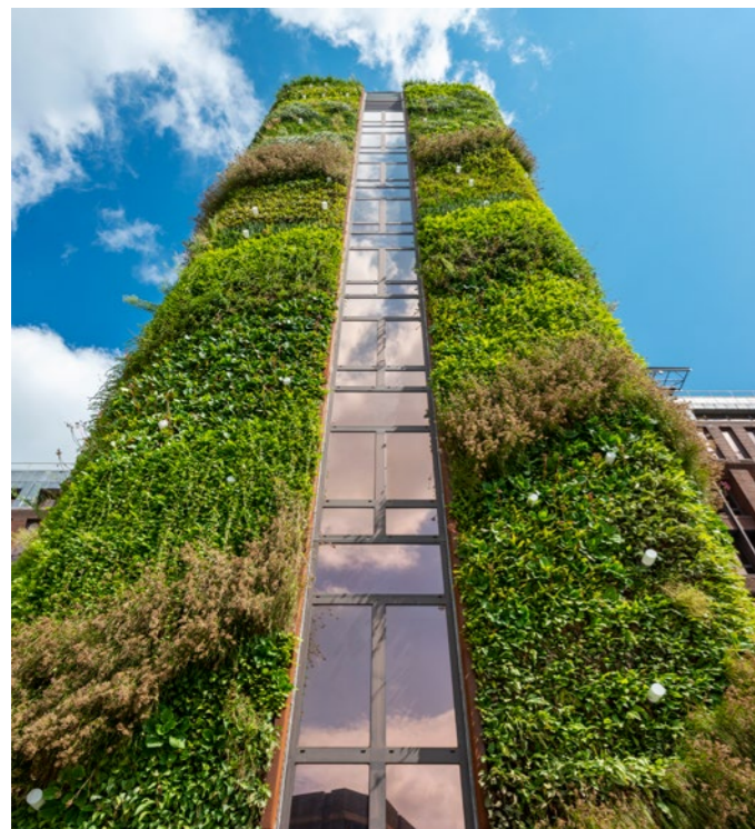
▲ Exterior living 'green' wall
