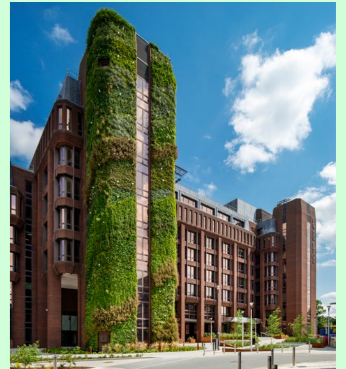
▲ Exterior living 'green' wall
