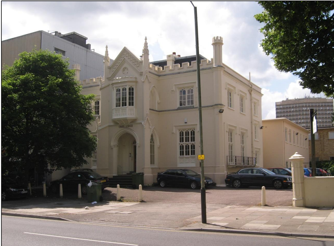
NB Old image – building undergoing refurbishment
